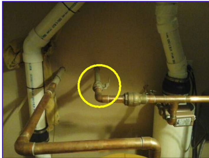
Water Heater supply shut off valve.
