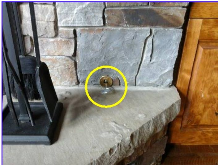
Gas log starter valve for fireplace. Turn clockwise to turn off.
