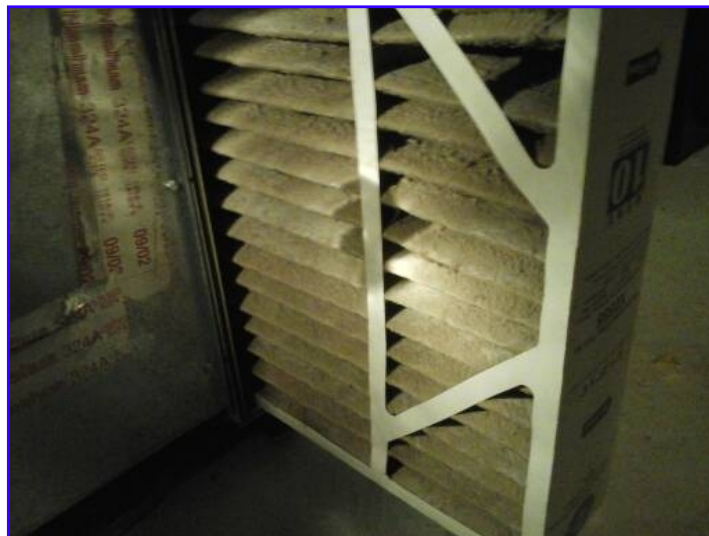
Replace dirty filter. 20x25x5, MERV 10 or better.
