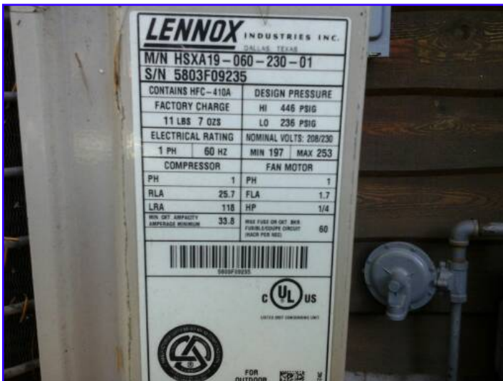
5 Ton capacity compressor.
