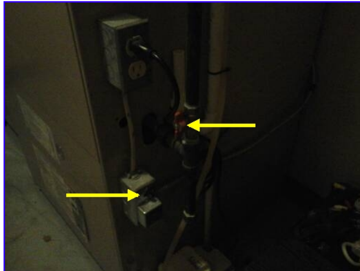
Gas shut off valve at top arrow, main furnace electric cut off switch at bottom arrow.
