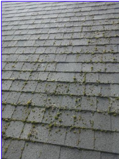
Moss on North side of roof.
