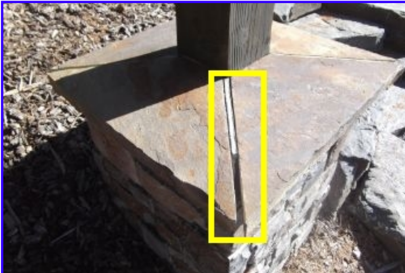
Cracked and missing grout around lower deck posts needs to be repaired.
