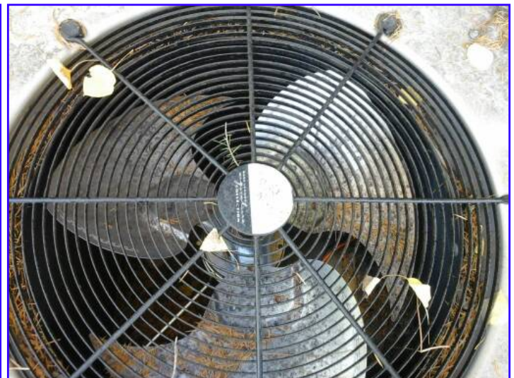
Clean pine needles and leaves from compressor housing.
