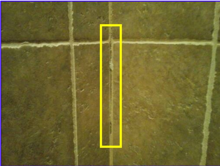
Seal or re-grout where required.
