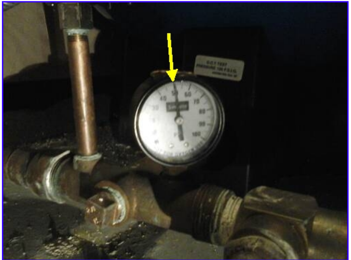
Pressure switch set to 50 psi.
