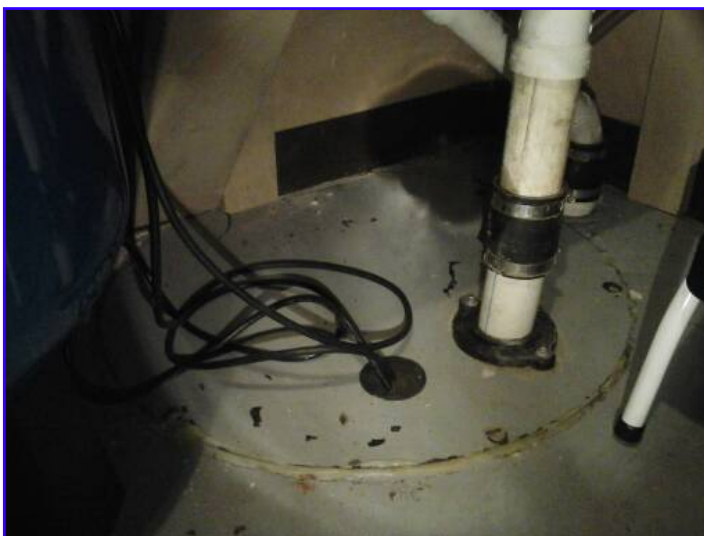
Sewage grinder/pump in basement mechanical room.
