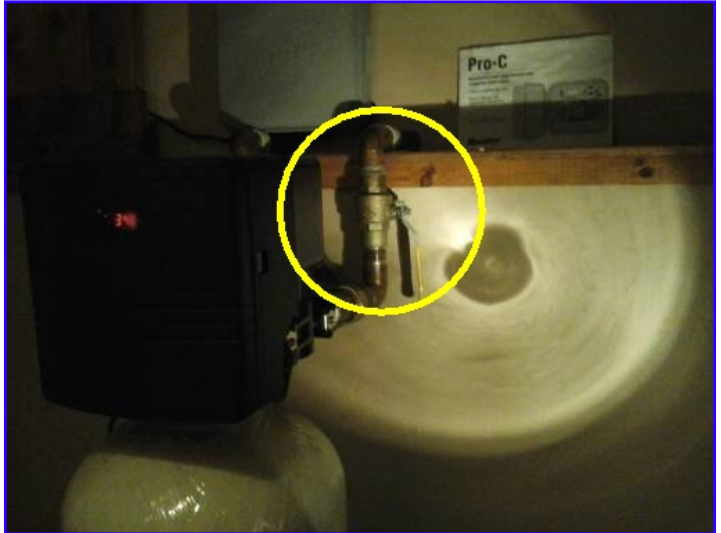
Main house water supply shut off valve in mechanical room.
