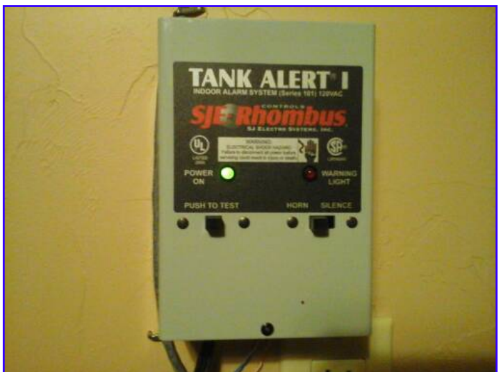
Septic alarm in mechanical room.
