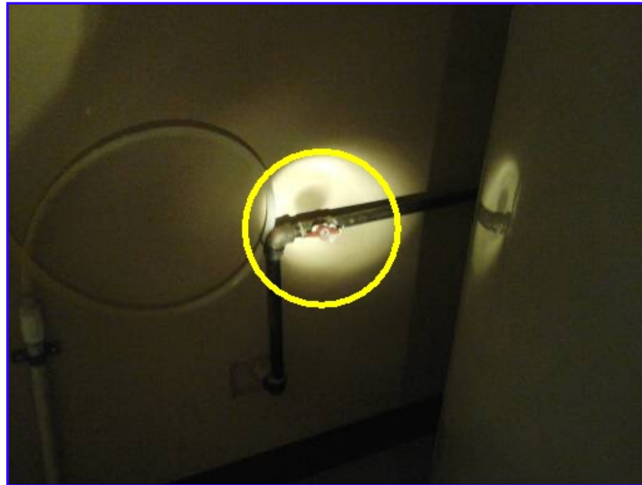
Water heater main gas shut off valve.
