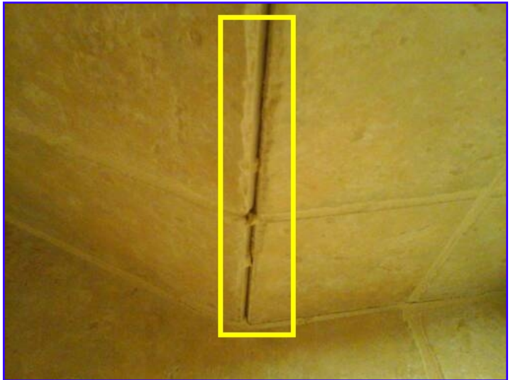
Seal or re-grout where required.
